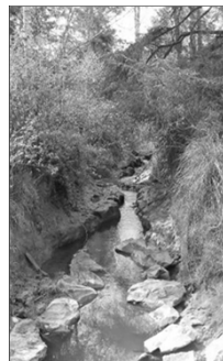
Incised channel upstream of culvert replacement
